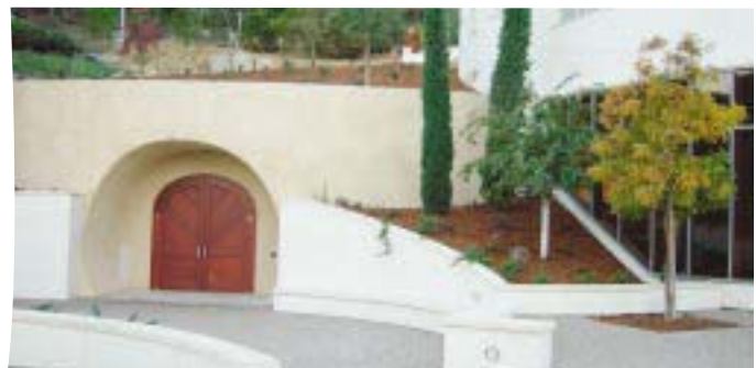
Behind these doors a pair of Capstone C60 microturbines spin natural gas into power, heat and cold.
