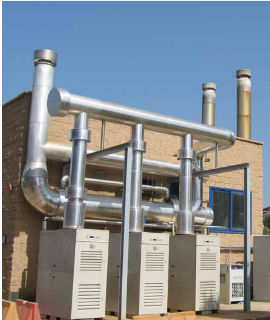
Three 60kW Capstone microturbines running on biogas generate heat and power at Edar de Rubi WWTP in Spain.
