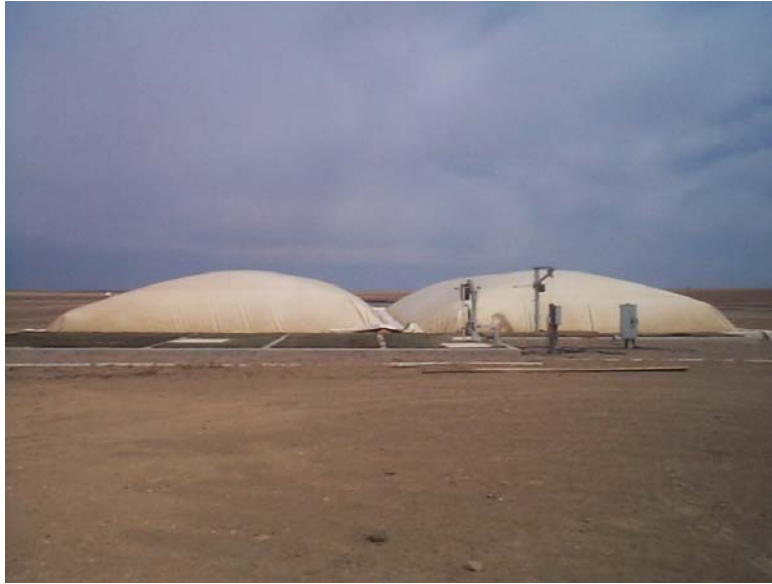
Figure 1-3. Colorado Pork Anaerobic Digester
