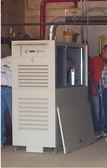
Capstone 30 kW Microturbine
